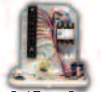
End Tower Box
